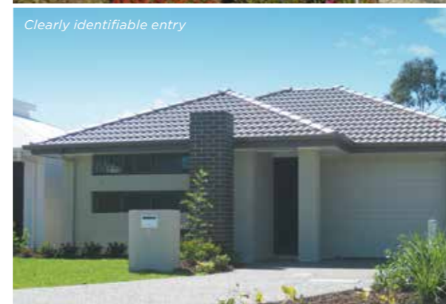
Articulation through windows and cladding
