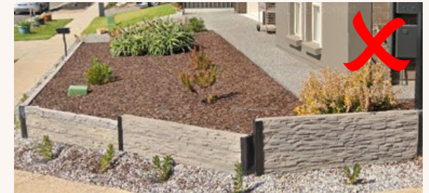
Sectional or sleeper retaining walls are not permitted where visible in public areas.
