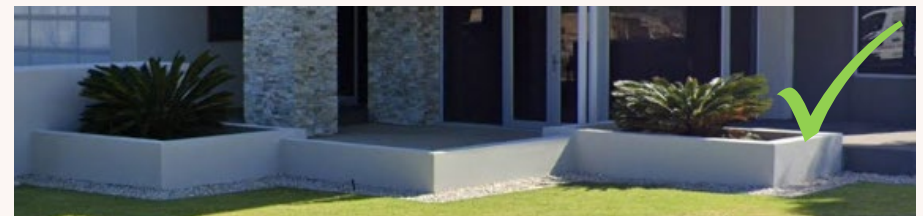
White rendered masonry retaining walls may also form landscape feature planters.
