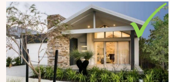
A highly articulated front façade including a feature verandah / porch, stone clad pillar and clerestory windows.
