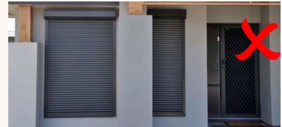
Security roller shutters and traditional lattice style security screen doors are not permitted.
