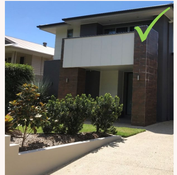
White rendered masonry retaining walls are acceptable.
