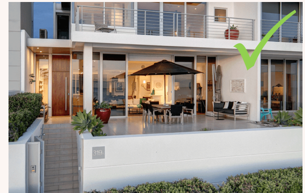
Seamless incorporation of an access gate into the retaining wall design, and beachfront outdoor area.
