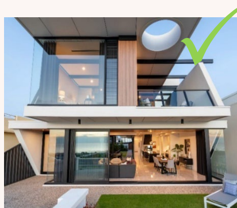
An example of nautical theming used in the façade design, combined with modern feature glazing and premium finishes.
