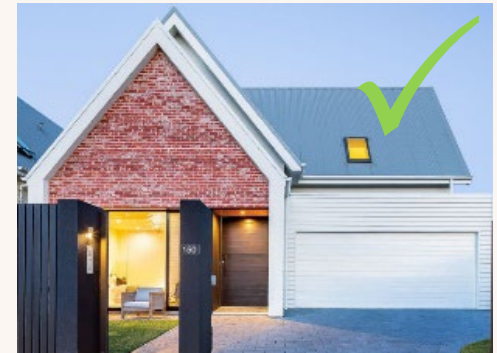
An example of a gable end roof style with decorative brick infill.
