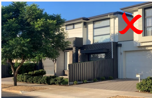
Side boundary fencing forward of the home needs to be open style, 1.2m high maximum.
