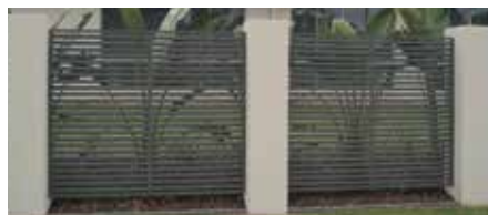
Street frontage/ secondary street frontage masonry fence
