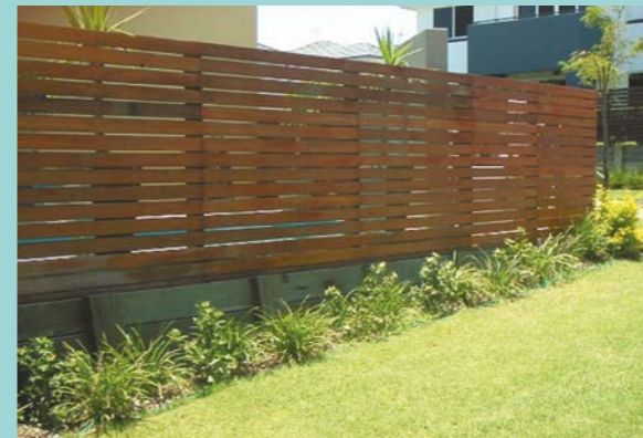
IMAGE 5 SECONDARY FRONTAGE/CORNER LOTS – EXAMPLE 1 For corner boundaries, stained or painted horizontal or vertical slat fencing. 1800mm in height measured from ground level, minimum 20% transparency (i.e. 22mm spacing between 90mm timber slats).
