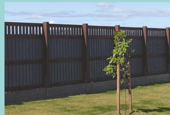
IMAGE 6 SECONDARY FRONTAGE/CORNER LOTS – EXAMPLE 2 For corner boundaries, stained or painted horizontal or vertical slat fencing. 1800mm in height, can be solid to 1500mm if openings are more than 50% transparent above 1500mm.
